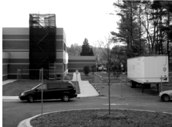
Work zone at back of CGES
